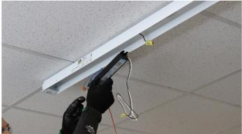
**Step Four:**Using tether cable (supplied), hang Retrofit tray from an existing hole in housing to be retrofit as seen below. Connect ground wire from LED Retrofit tray to the fixture housing by connecting to the existing
