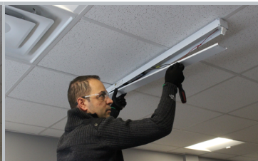
Step Two: Remove Ballast Cover and Recycle/Discard
