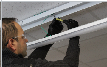
Step Five: Connect LED Driver Disconnect to Main power. Raise LED retrofit tray and center equally from end to end. Secure in place using the 4 TEK self-drilling screws provided (2 screws for each end).
