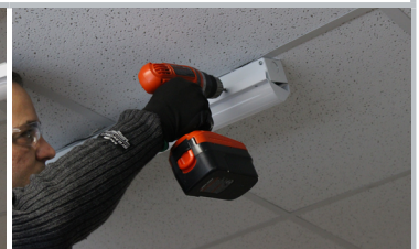
Step Five: Connect LED Driver Disconnect to Main power. Raise LED retrofit tray and center equally from end to end. Secure in place using the 4 TEK self-drilling screws provided (2 screws for each end).
